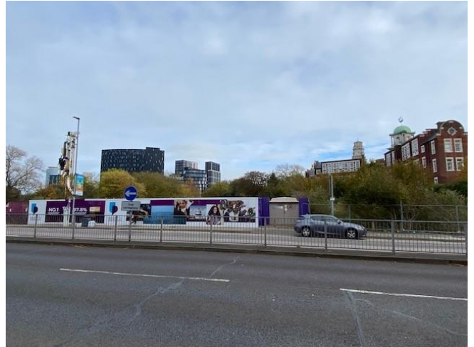
Photo 4: Looking east Anglesea Road
